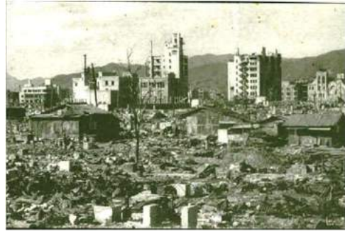
The Damage of Reinforced Concrete Buildings in 1945
